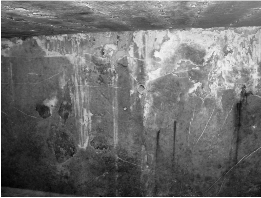
Figure 11. Rust stains and traces of calcium leakage on the side of a prefabricated vertical plate element.
